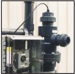
High Output UV Sterilizer is sized to the system's water flow rate and UV exposure requirements
