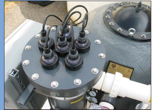
Watertight Electrical End of HO ML UV Sterilizer
