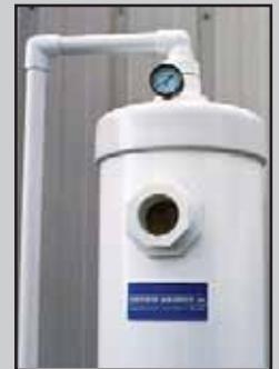
Pressure Gauge Assembly
